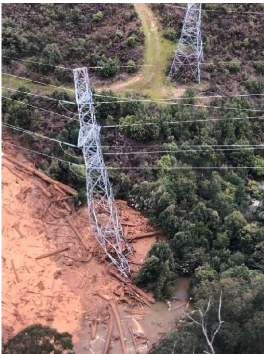
Figure 1 Photograph of double circuit strain tower damaged by landslide
