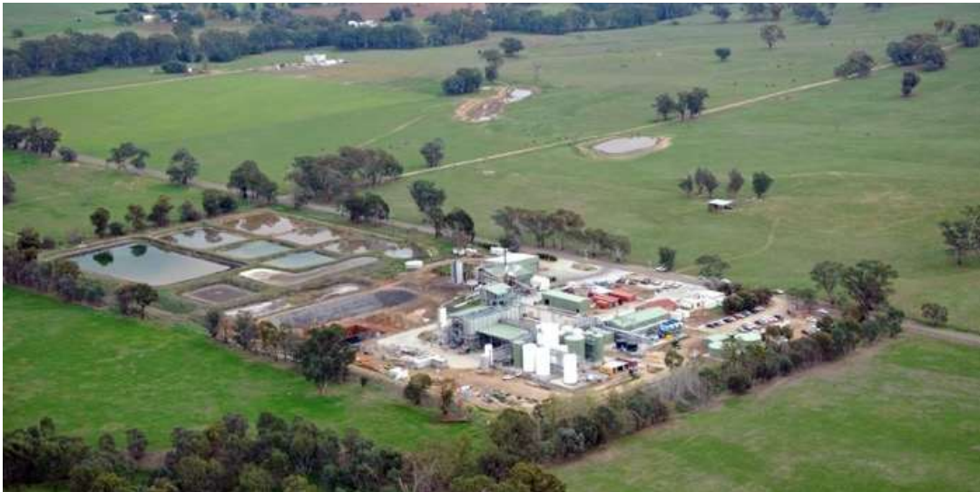
Figure 4-17 Just Biodiesel / refuelling solutions biodiesel plant, Barnawatha
