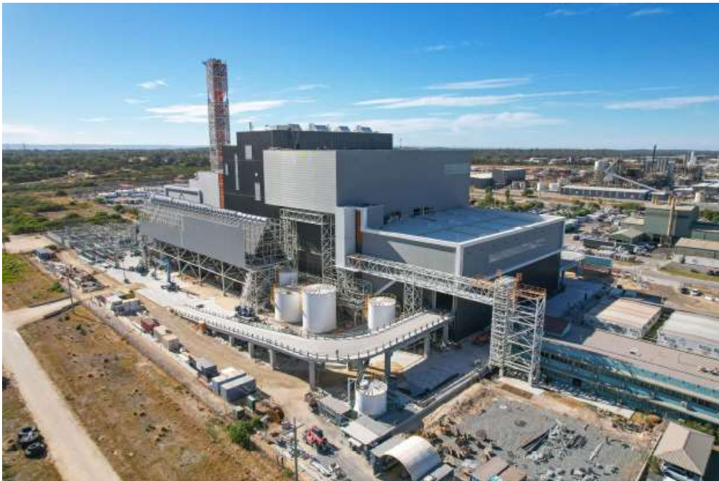
Figure 4-19 Kwinana Waste-to-Energy project, Kwinana WA
