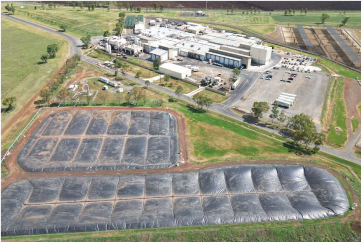
Figure 4-6 JBS Australia and Energy360 bioenergy system, Oakey Queensland
