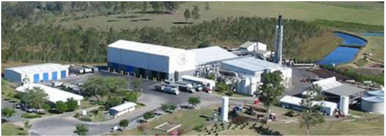
Figure 4-7 AJ Bush's Beaudesert biogas recovery plant in Queensland
