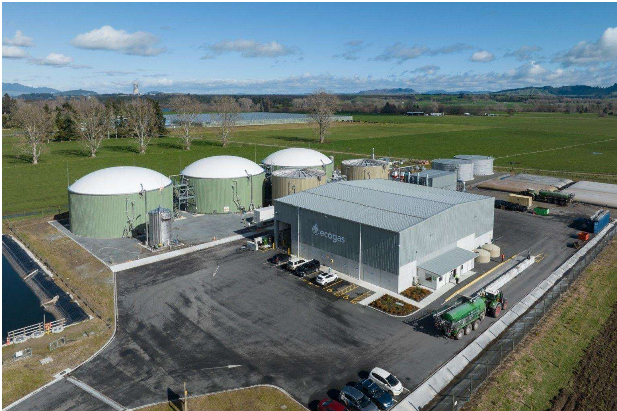
Figure 4-5 Ecogas's Reporoa organics processing facility, New Zealand
