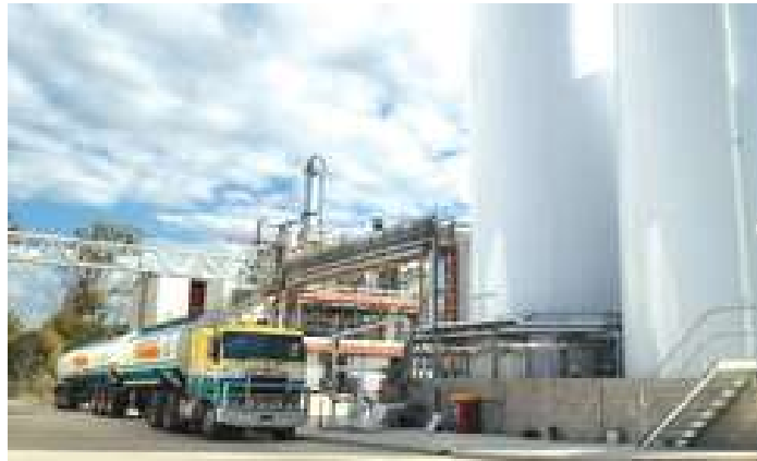
Figure 4-18 Ecotech Biodiesel plant, Narangba, Queensland
