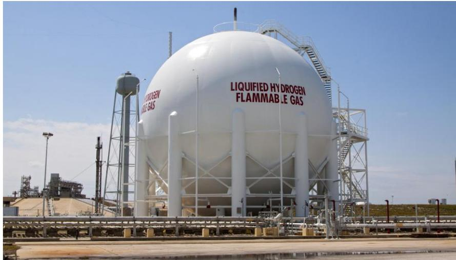
Figure 28: Liquid hydrogen storage vessel | Source: National Aeronautics and Space Administration (2015)
