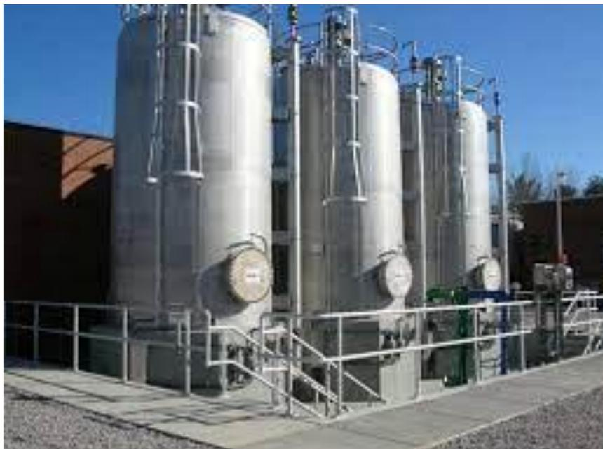
Figure 27: Above ground methanol storage tank | Source: Methanol Institute (2023)
