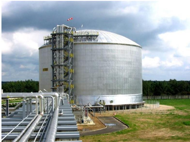
Figure 26: 15,000 tonne liquid ammonia tank | Source: thyssenkrupp Uhde
