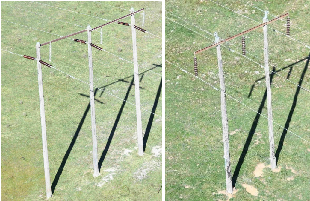
Figure 2-2 Line 977/1 tension wood pole structure (lefthand side) and suspension wood pole structure (righthand side)
